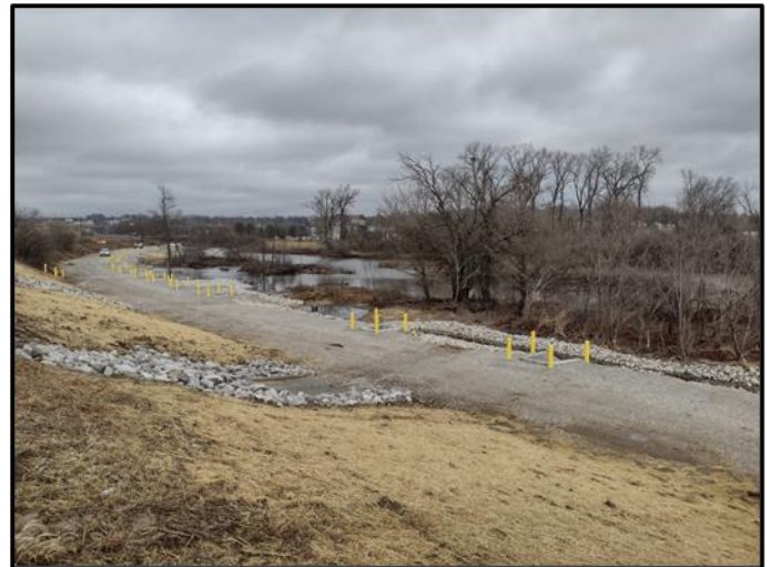
Figure 1: Reach 1 Construction Complete
